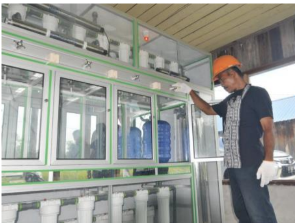
Fasilitas depot air minum WSS Saliki.
