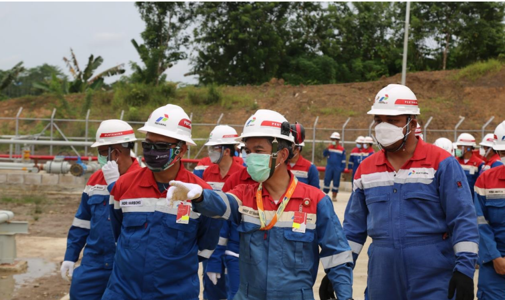
Management Walkthrough General Manager Zona 9 ke lokasi proyek New Samberah Oil Plant, 22 September 2021
