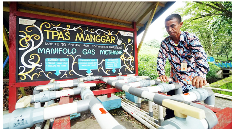
Monitoring Program Wasteco di TPAS Manggar.
